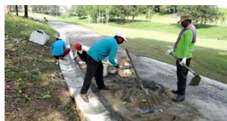
STEP 5 Applying cement on all joints
