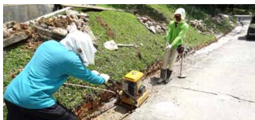
STEP 3 Compacting the spoon drains
