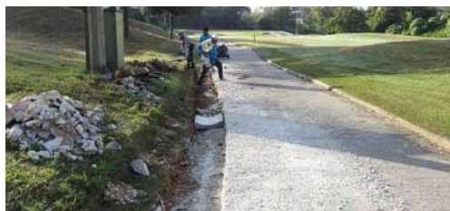
STEP 1 Hammer-breaking the old v-drains
